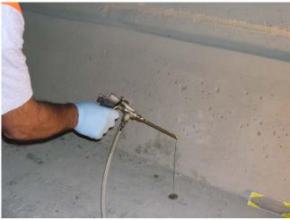
At this stage plug the first tube and repeat the procedure upwards until completing the whole job. The pump pressures have to be determined on site since they can vary according to the size or depth of the crack.
