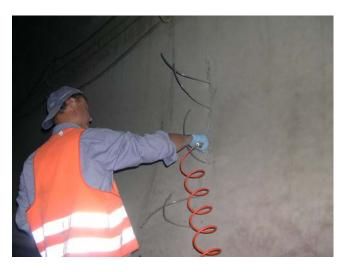
When the seals are set (after approx. 24 hours), connect the pump to the lowest tube and begin injecting, gradually increasing the pressure. If resin leaks from the next tube above then the crack being treated has been filled.
