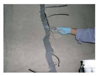
Remove any loose or crumbling parts and blow out any dust with compressed air. Then fit copper tubes, having an 8-mm section, in the holes, seal the cracks and fix the injection tubes with the adhesive MasterInject 1360.
